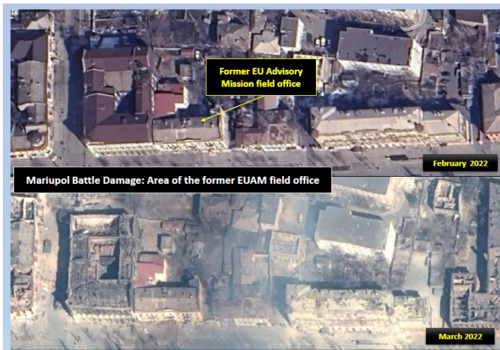
Daños en la EU Advisory Mission Field Office
